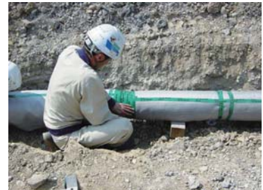
Photo: Installation of protective
