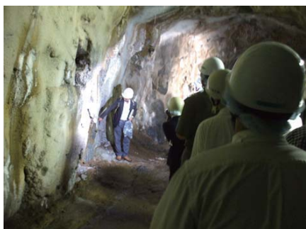
Photo: Researchers checked hardness of rock at power station
