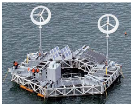
Figure 2. A floating structure equipped with offshore wind power generation facilities installed in Hakata bay(December 2011)
