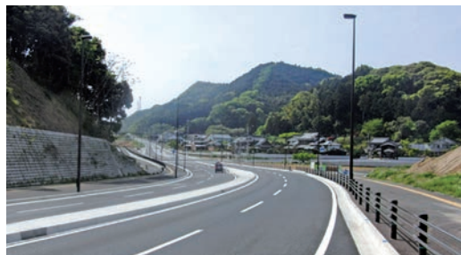
Picture: the newly constructed road (toward Sakurai)
