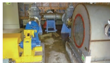
Picture: The power generation device set in Shiraito-no-taki Fureai-no-sato Cross-flow waterwheel + Adjustable three-phase synchronized power generator (left: 5kW) & Pelton wheel + Outer rotor power generator (right: 10kW)
